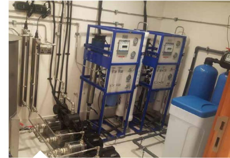
Under our Water Division, SE Dubai installed and commissioned a state-of-art water treatment system at one of the leading hospitals in UAE: Al Zahraa Hospital (Sharjah). The system produces 3000 Gallons/day of ultra-pure water for kidney dialysis purposes – a complete desalination, disinfection & recirculation system that complies with the highest quality standards of water for medical purposes.
