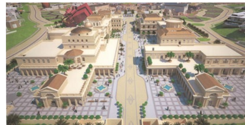
GALLERIES LAFAYETTE AT KATARA PLAZA We have been awarded the loose and fixed furniture contract by Ali Bin Ali Establishment in May 2017 which will be completed and handed over to the client by end February 2018.
